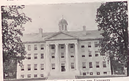
SOUTH BUILDING—IN WHICH ARE LOCATED THE UNIVERSITY ADMINISTRATIVE OFFICES
